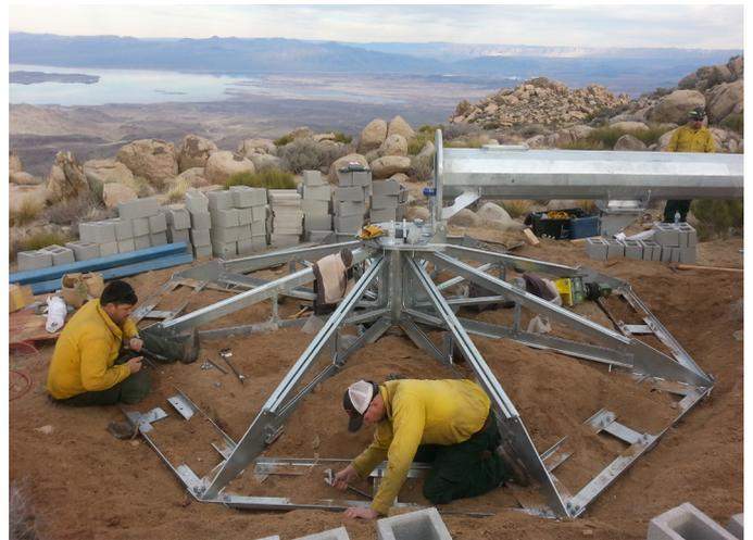
Example images of the Ground mounted (AFS) foundation which is ideal for remote or temporary installations
